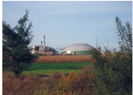
The largest dairy farm in Spain operates one of only 32 agricultural biogas plants in the country with slurry from 2500 cows. The digestate is dried and sold as fertiliser for organic agriculture. Photo: STUDIA
