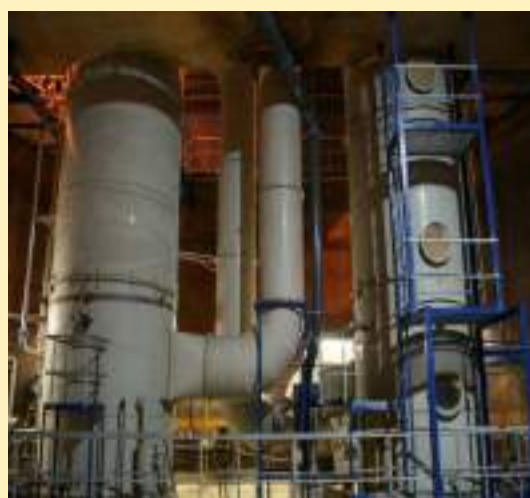
Picture (Courtesy of VEAS). Nitrogen recovery at VEAS wastewater treatment plant in Oslo (Norway). Right is the ammonia stripping tower, and left the acid absorption tower.
